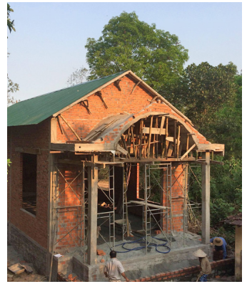
Church Almost Finished
